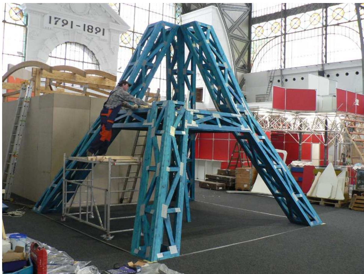
Assembly of the tower at Prague Fair grounds
