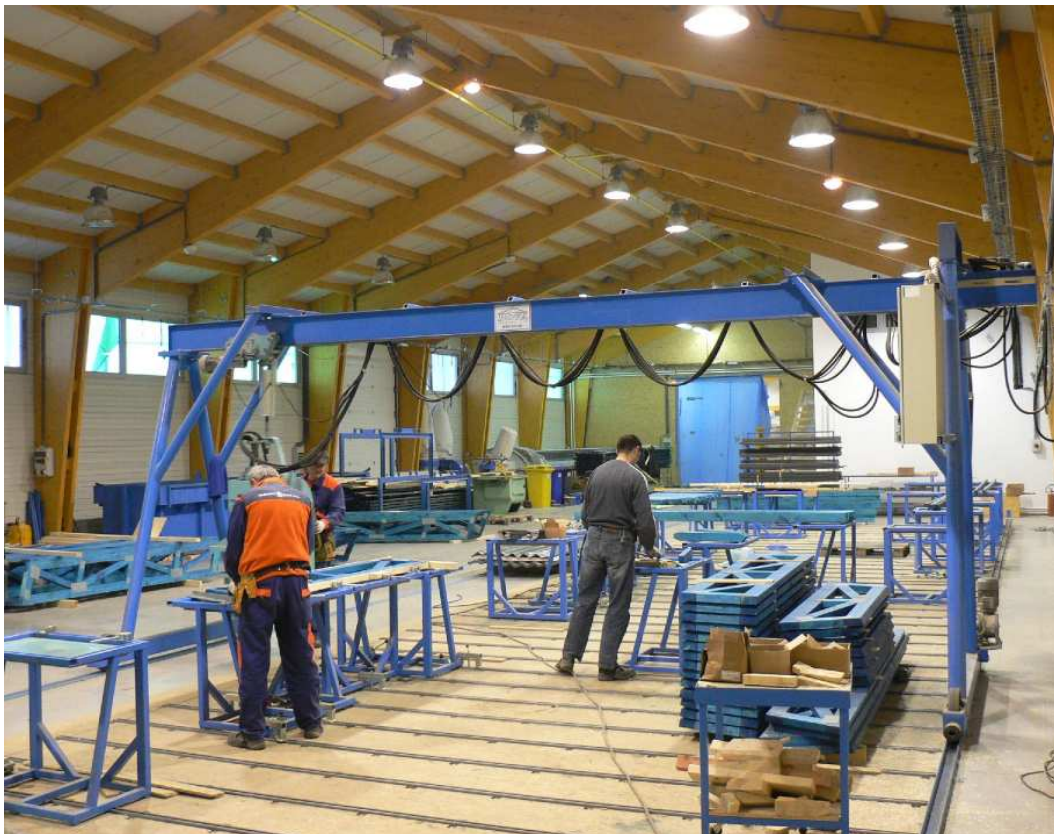
Production of the tower trusses in a new fabrication hall of the company
